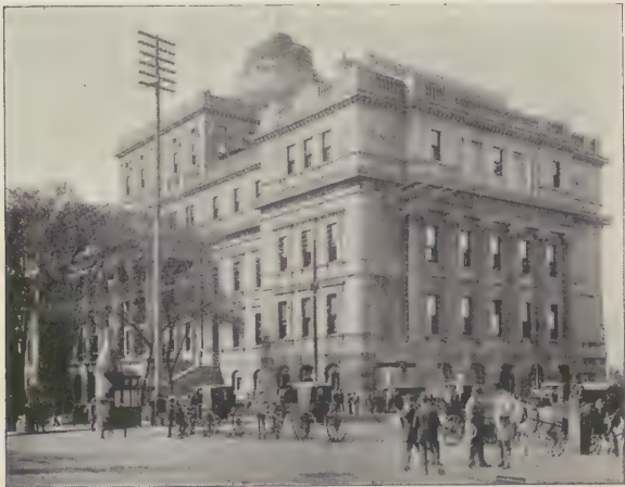
COURT HOUSE, MONTREAL.
